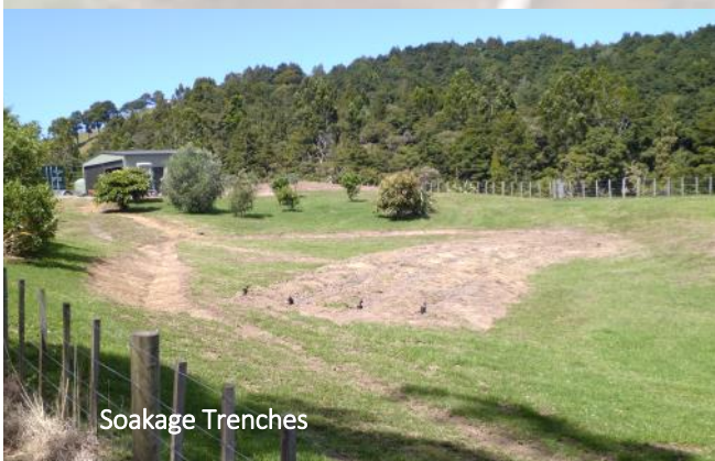
Soakage Beds during installation
