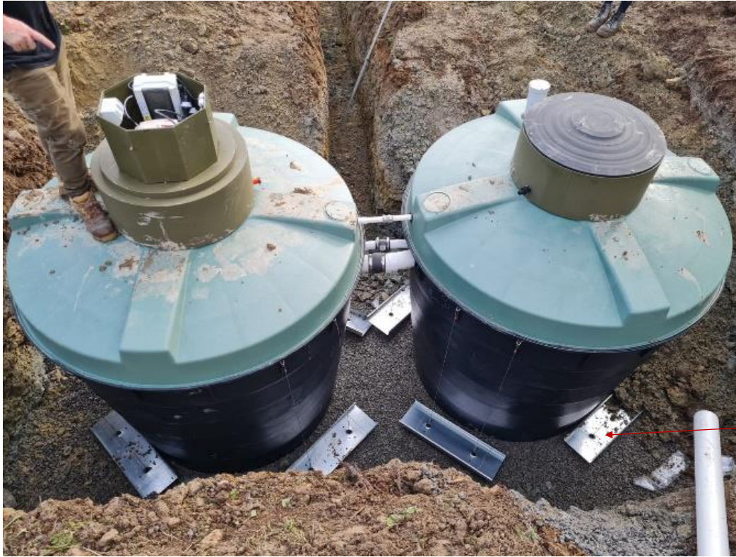
C. 4 x Uplift restraint plates tied to each tank
