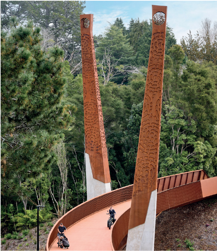
Left and above: Both steel masts, or taurapa, feature a twin-skinned steel form, with intricate Māori artwork laser-cut into the outer skin. Steel enabled the refined form envisioned by the architects, while meeting the bridge's structural demands.
